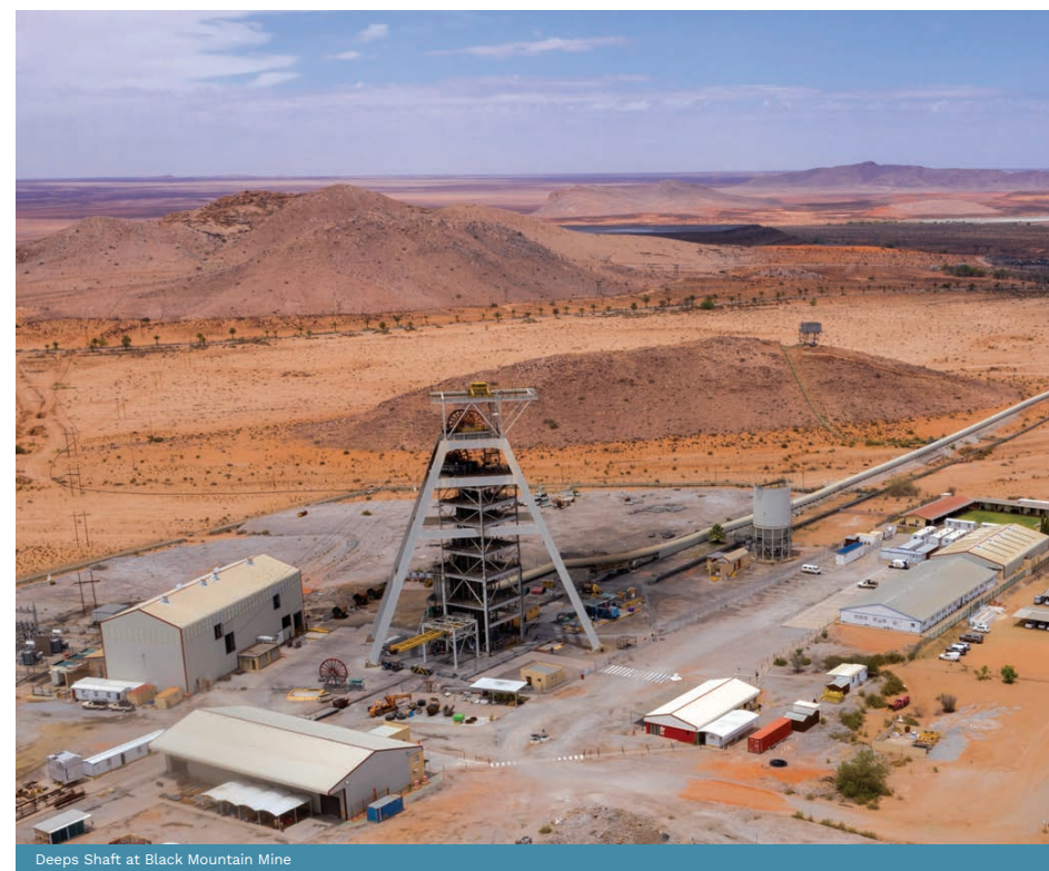
Deeps Shaft at Black Mountain Mine
