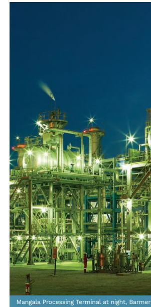
Mangala Processing Terminal at night, Barmer
