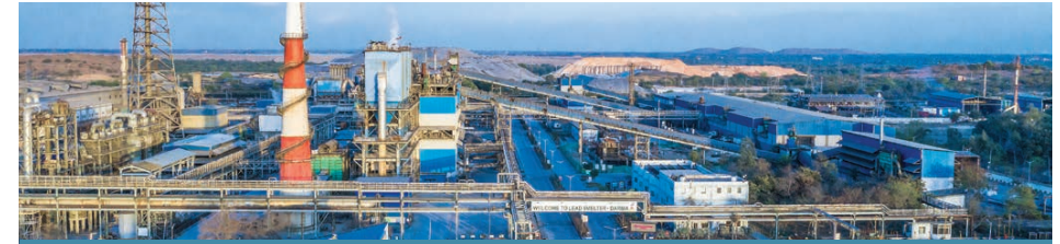
Dariba Lead Smelting Complex, HZL
