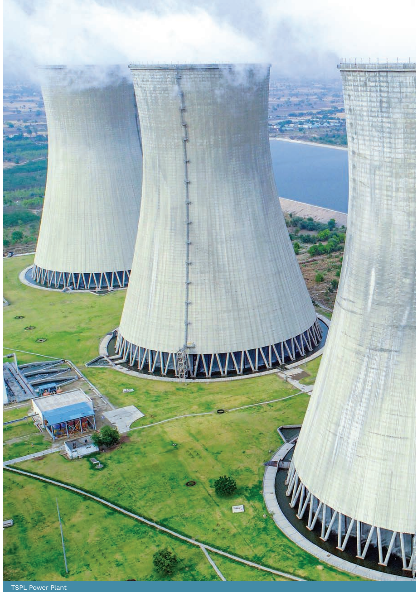
TSPL Power Plant
