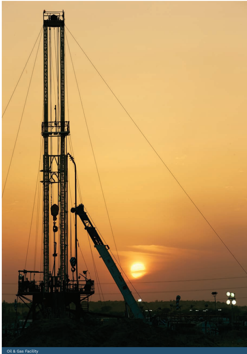
Oil & Gas Facility
