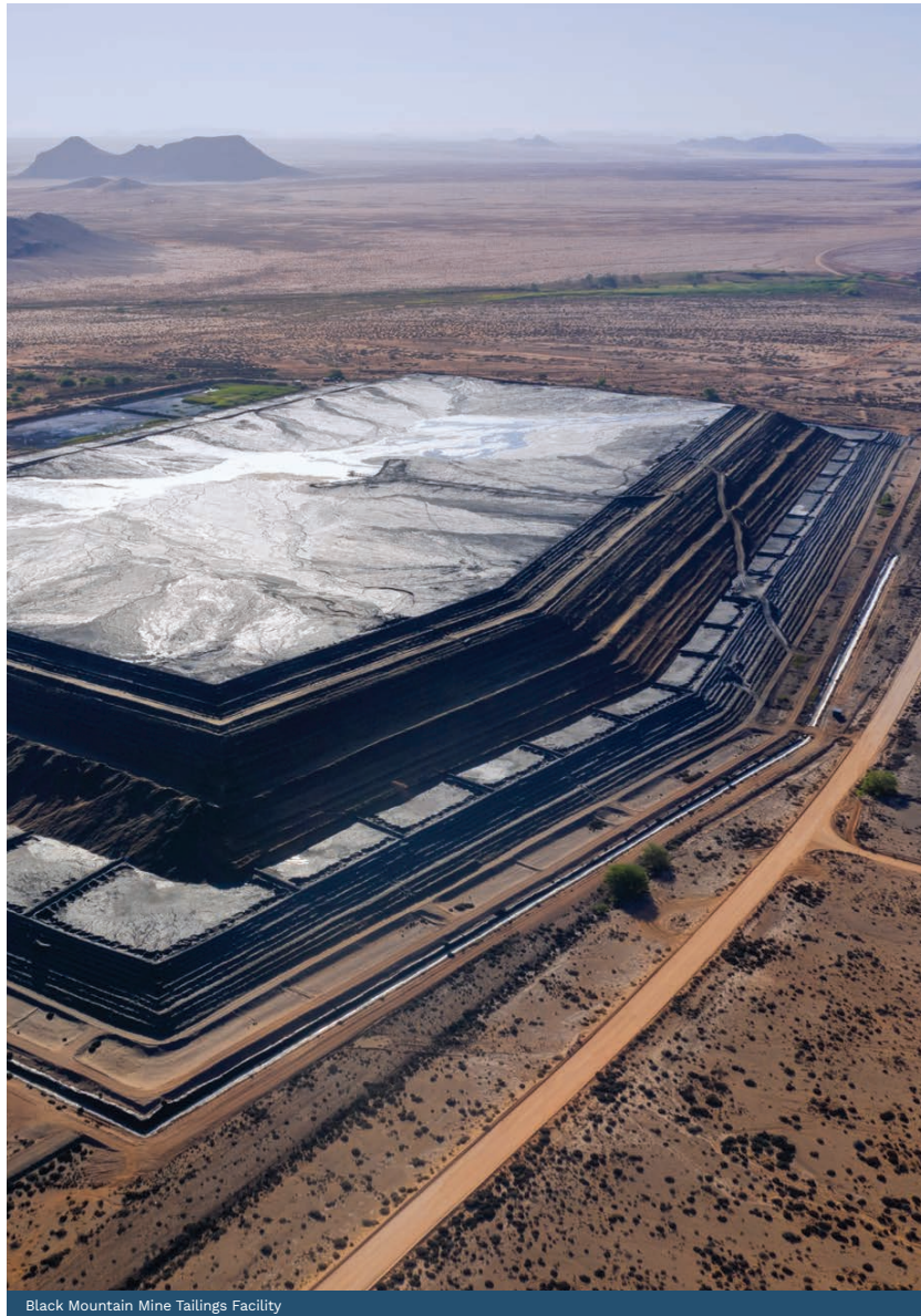
Black Mountain Mine Tailings Facility
