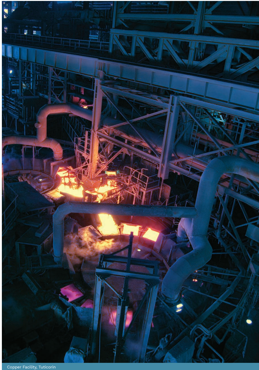
Copper Facility, Tuticorin
