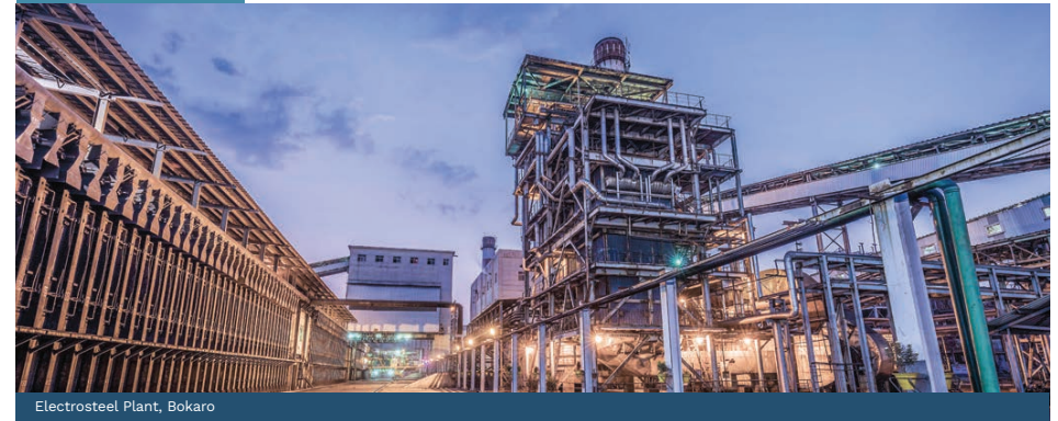
Electrosteel Plant, Bokaro
