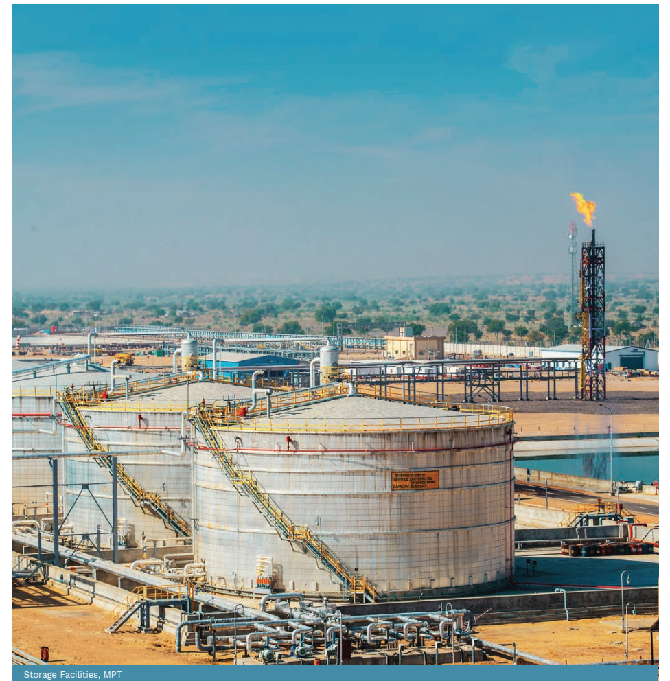
Storage Facilities, MPT
