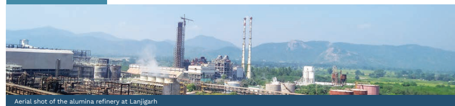
Aerial shot of the alumina refinery at Lanjigarh
