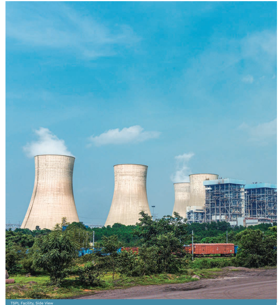
TSPL Facility, Side View
