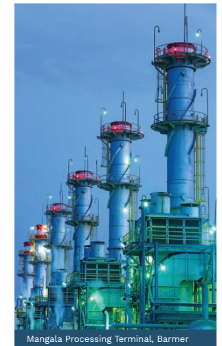
Mangala Processing Terminal, Barmer
