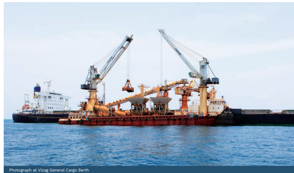
Photograph at Vizag General Cargo Berth
