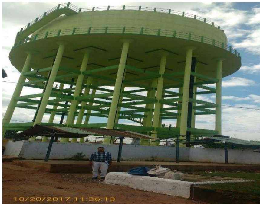
FIGURE-28 NEWLY CONSTRUCTED WATER TANK IN WARD NUMBER 40
