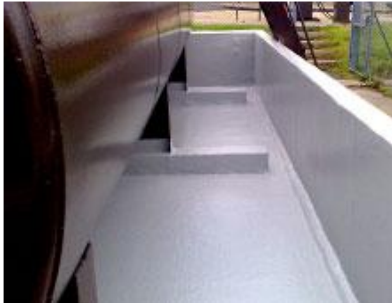
Example of a bulk storage tank within a bund
