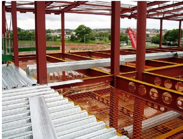
Example of safety nets applied at the “leading edge” on a construction project.
