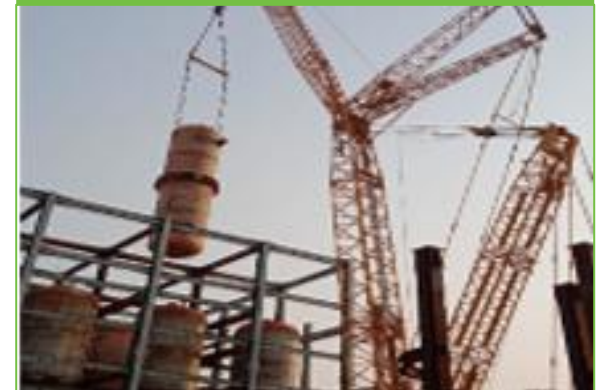
Digestion Vessel erection
