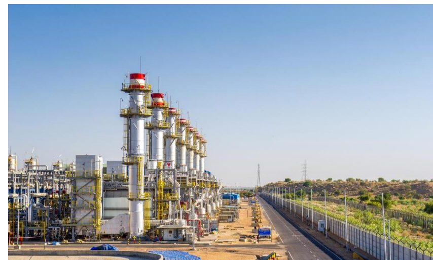
Rajasthan: Captive Power Plant - Steam Generation
