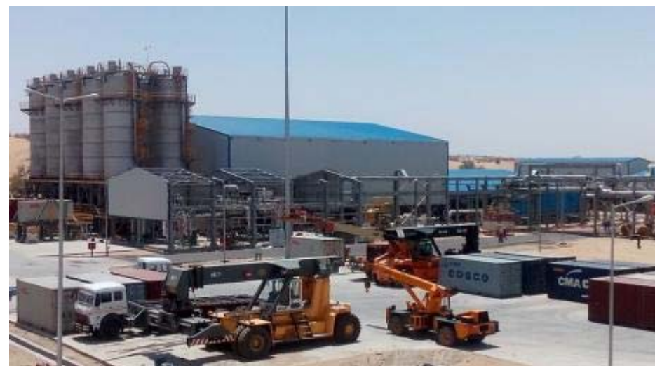
Central Polymer Facility, Rajasthan
