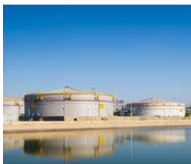
Left: Rajasthan: Mangala Processing Terminal Right: Rajasthan: Polymer Storage Silos
