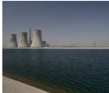
Left: Power plant
